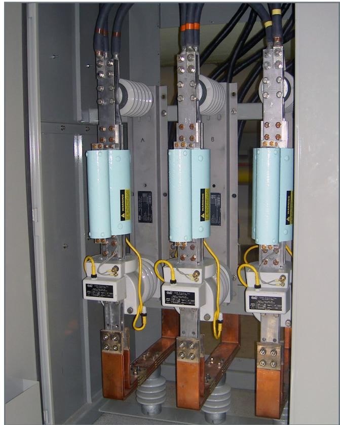
▲ CLiP protecting a methane fueled co-generators in a sewage treatment plant.
