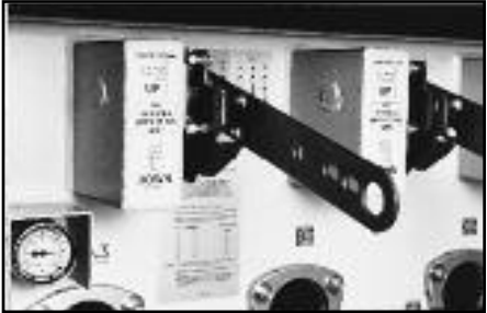
▲ Single phase interrupter operating handles.
