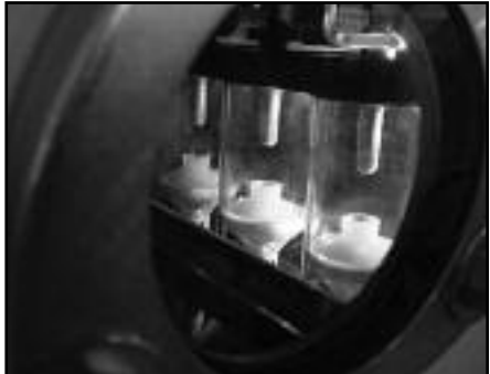
▲ Load break switch visible break.
