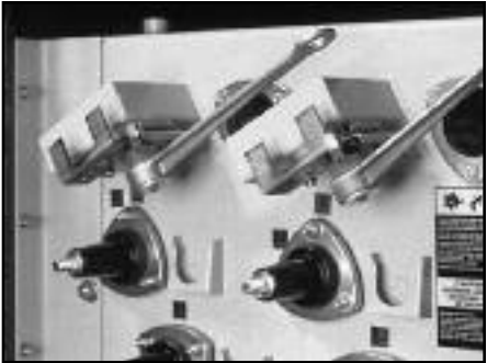
▲ Hookstick operable load break handle.
