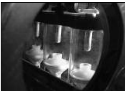
▲ Three phase visible position of contacts.
